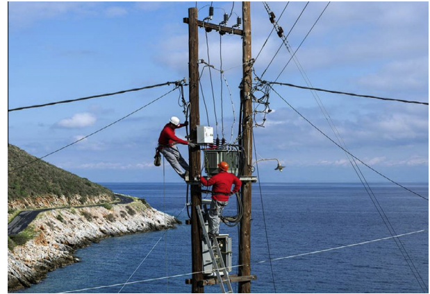
Fig. 3. Rayvoss protection system being installed at a distribution transformer of PPC.
